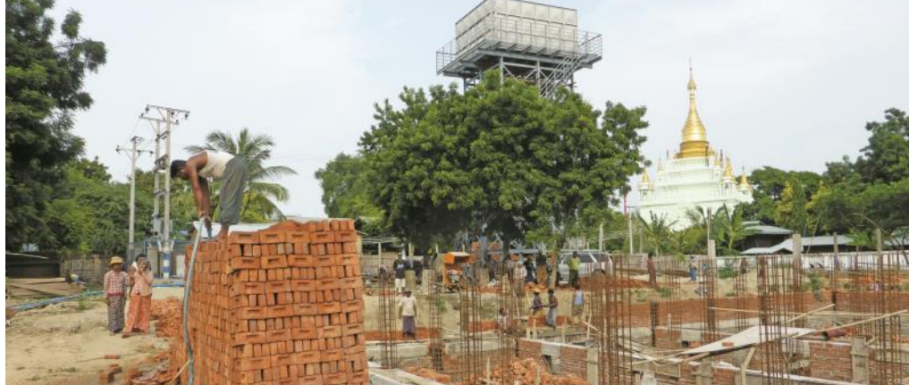
Construction of a water production facility in Amarapura Township
